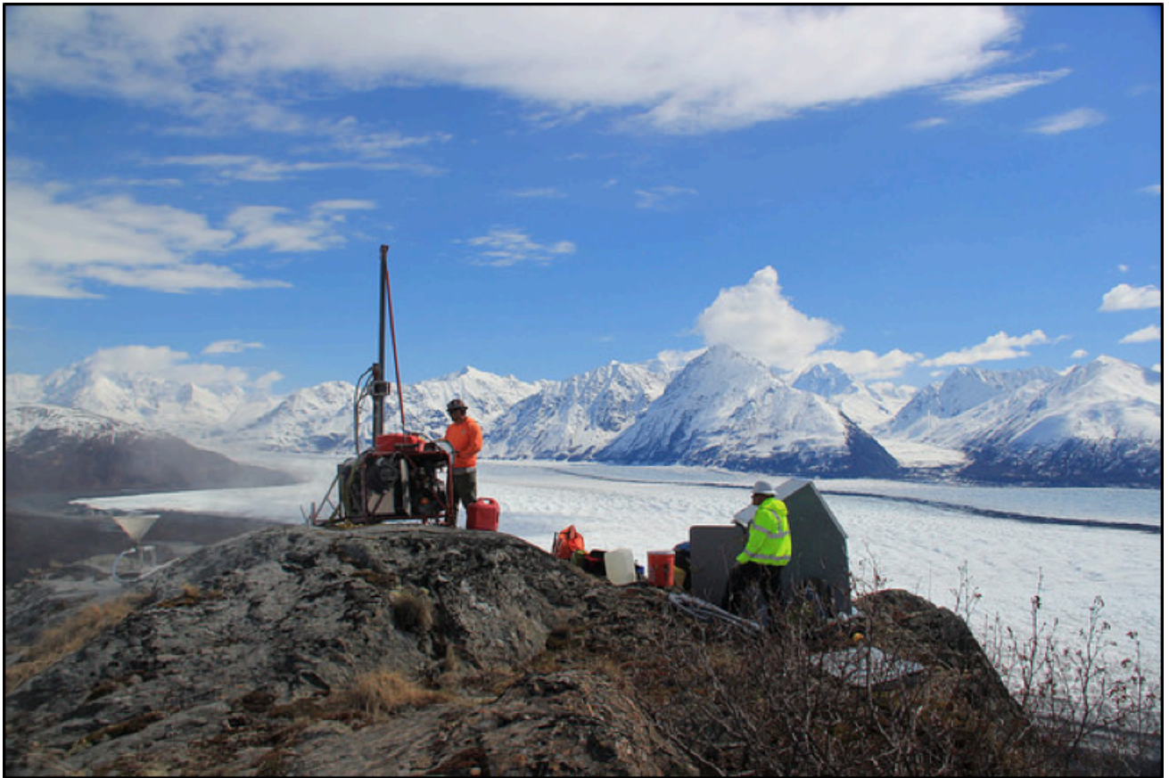
Installation of a Transportable Array station in Alaska (2015)
