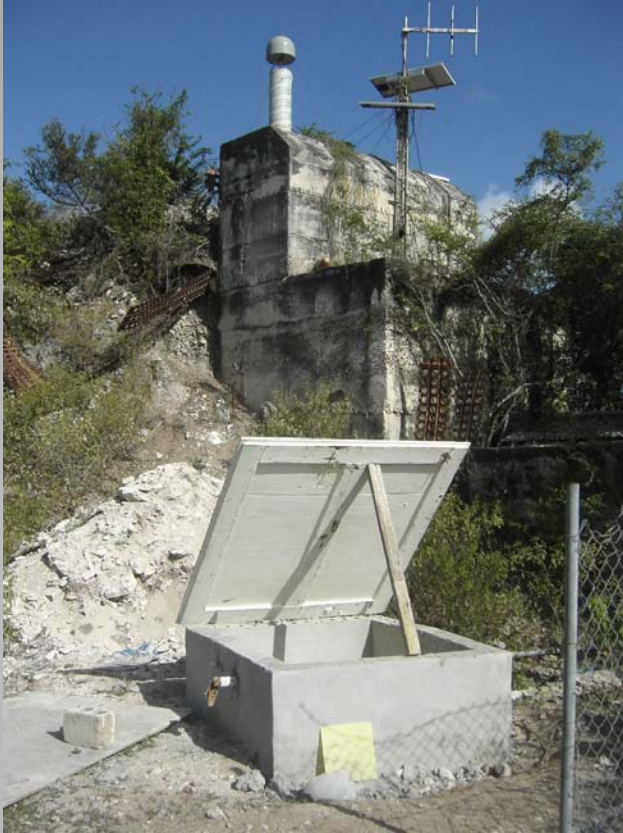
Section of the Aneгада Seismic Station: GPS and Sensor containment unit
