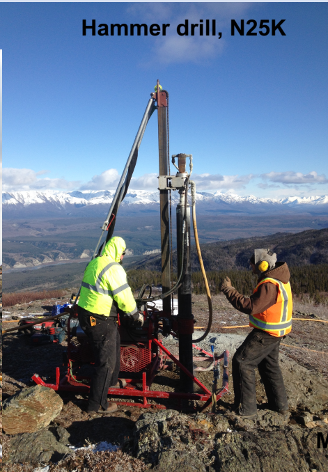
Hammer Drilling, AK.SCRK
