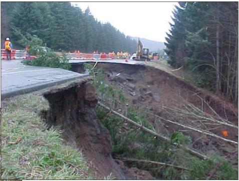
US Highway 101 landslide. The curved headscarp of the landslide is 24 m wide
