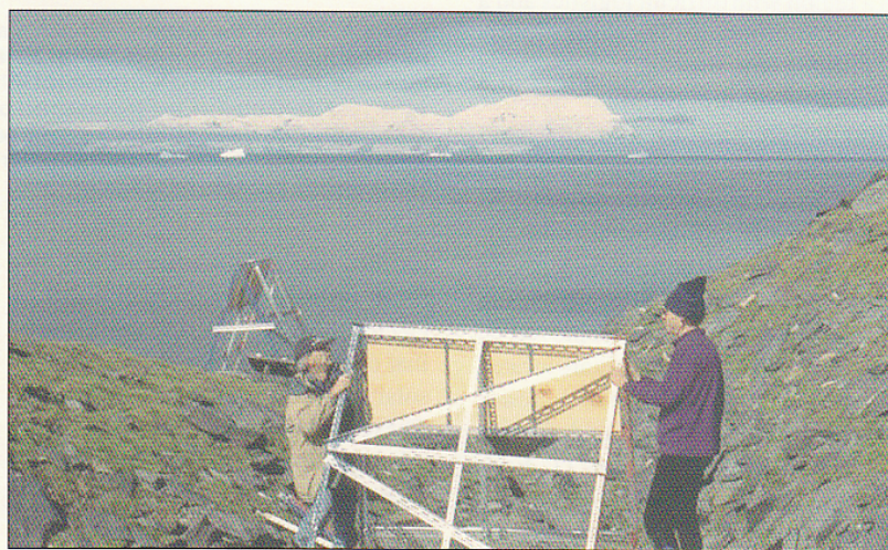
Figure 3. Patrick Shore (Washington University) and Paul Friberg (Lamont PASSCAL Instrument Center) install banks of solar panels at Elephant Island, South Shetland Islands. The glaciers of Clarence Island tower in the background. The Elephant Island station ran unattended for nearly one year over the Antarctic winter.
