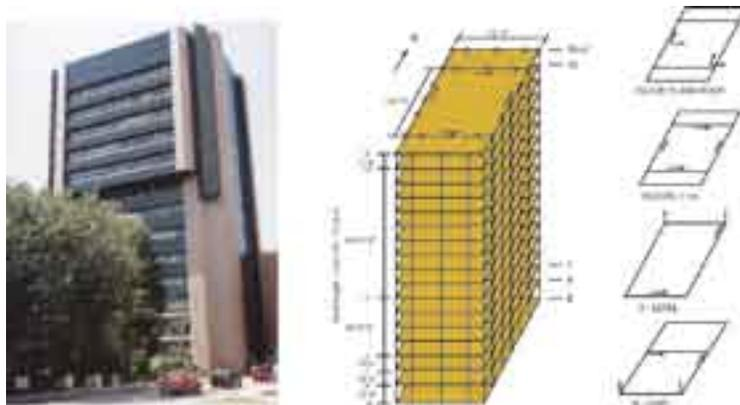
Figure 1. (left) Photo of Factor building and (right) diagram of sensor locations. Arrows show polarities of sensors on each floor. The 72 channels of building data can presently be viewed on the web at [teren.ess.ucla.edu:5813](http://teren.ess.ucla.edu:5813) (password: seismo) in real time.
