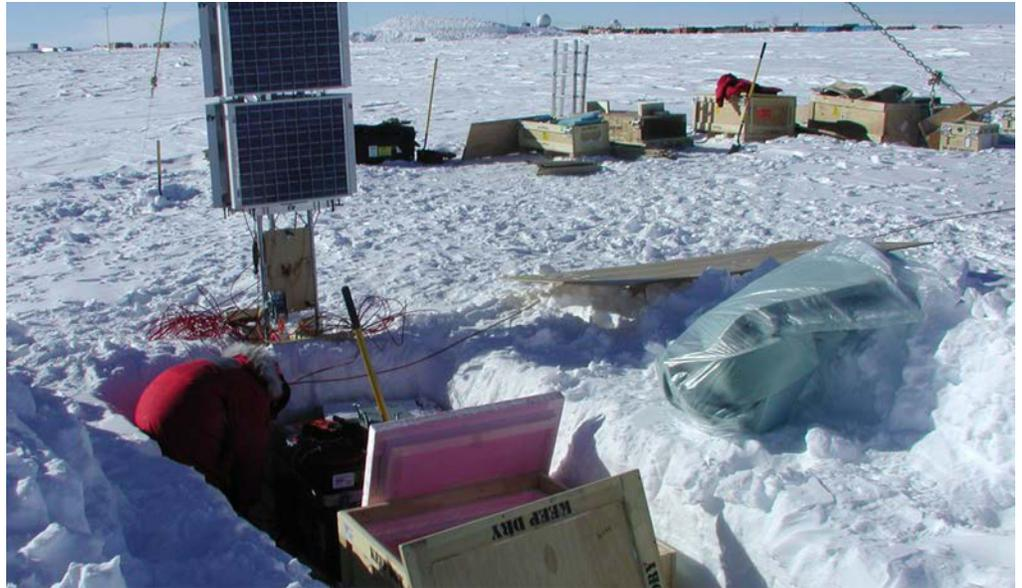
**FIGURE 8.** Installation of a low power magnetometer system at the South Pole station for testing. Stations such as South Pole serve as important testbeds where autonomous equipment can be debugged prior to deployment in remote locations.
