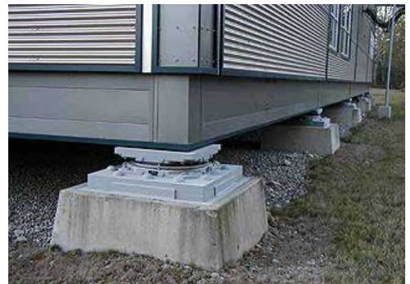
Base isolators at the Washington Emergency Management Division building. Photo courtesy of Washington State Military Department Emergency Management Division
